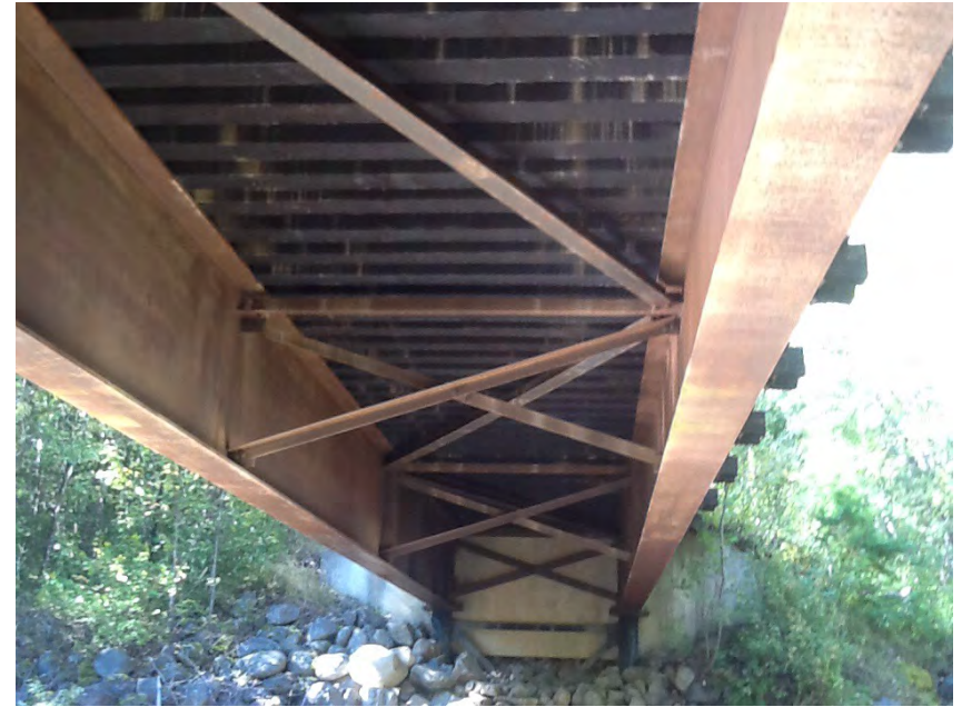
Underside of bridge
