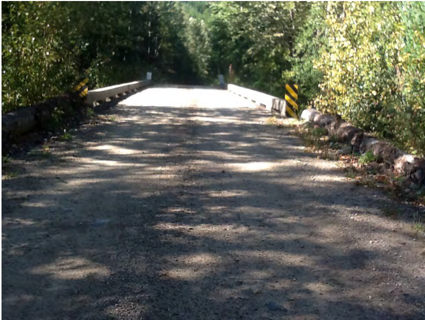
Right approach facing structure
