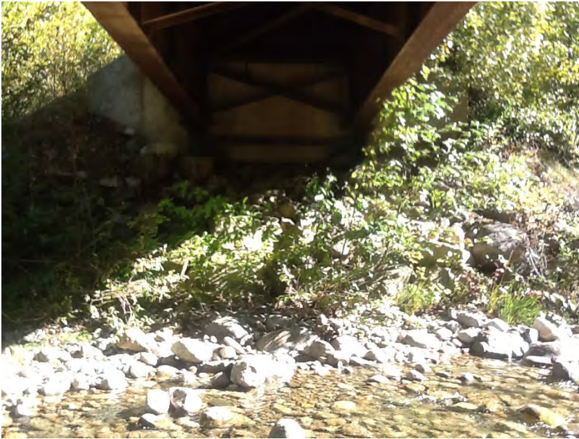
Right Bank Abutment when facing downstream
