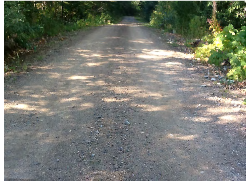
Left approach facing away from structure
