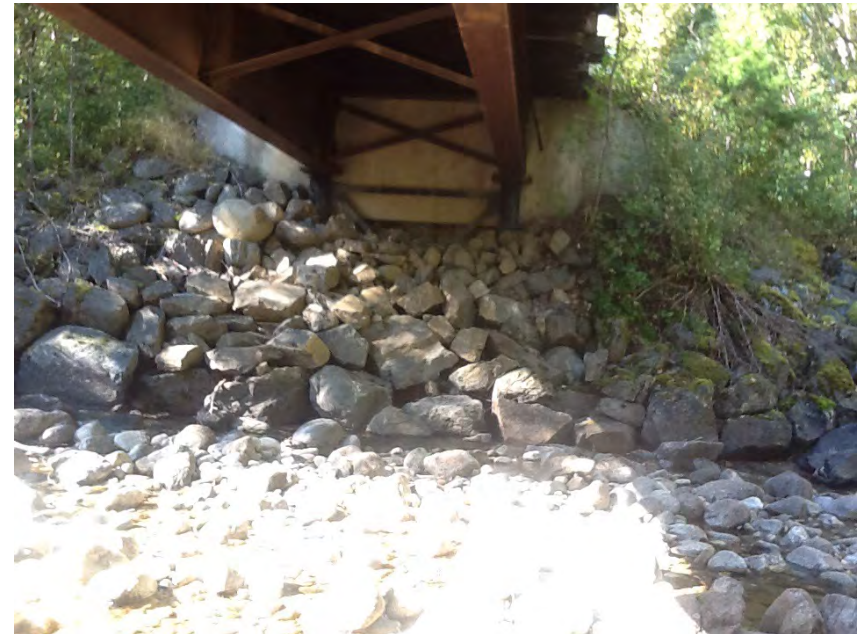
Left Bank Abutment when facing downstream
